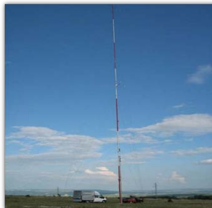
60m meteorological mast in Bulgaria
