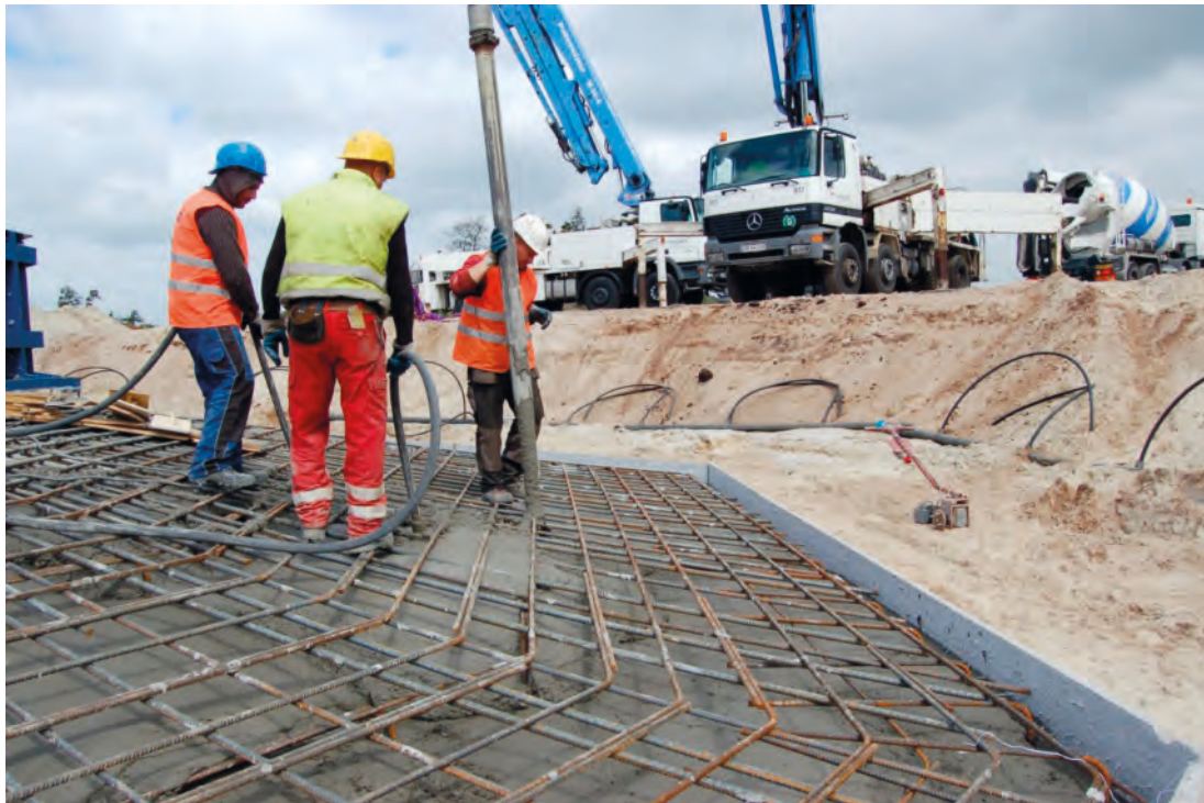
European Energy – concreting foundation in Danish wind park
