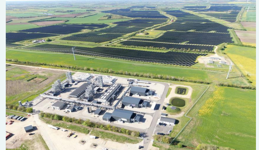
Kassø PtX – world's first large-scale commercial e-methanol facility
